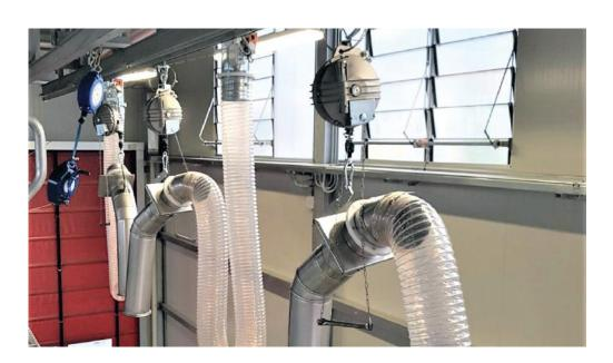
Both systems feed devices, made to flow in a line parallel to that of the washing heads, with which the hot air, filtered according to the standards set by food and chemical companies, is introduced into the tank.
