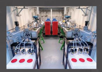
If rooms for the installation of the thermal and pumping plant are not available, OMZ prepares 20-foot containers, for the purpose, completely insulated, class 0 of fire resistance, complete with lighting system and ventilation outlets.
